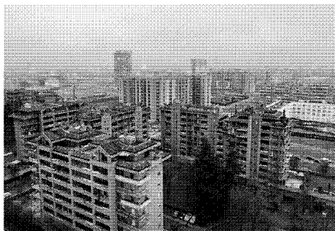
■ "THE MILAN MODEL" HAS MEANT A RUTHLESS REAL ESTATE DEVELOPMENT OF THE CITY. AERIAL VIEW OF THE PERIPHERAL NEIGHBOURHOOD OF QUARTIERE ADRIANO, IN THE NORTH OF MILAN.
